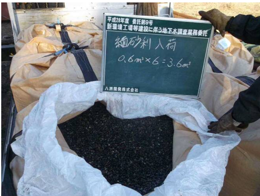
材料入荷 緬砂利 0.6\text{m}^3 \times 6 = 3.6\text{m}^3
