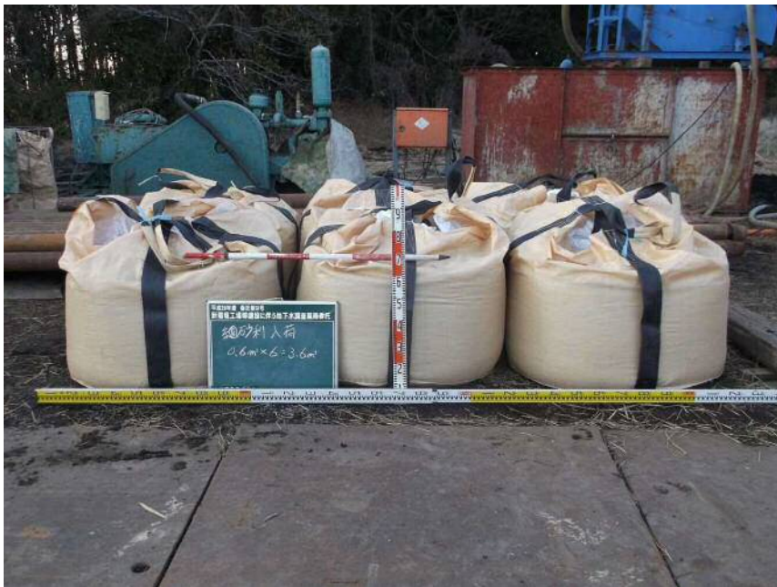
材料入荷 緬砂利 0.6\text{m}^3 \times 6 = 3.6\text{m}^3
